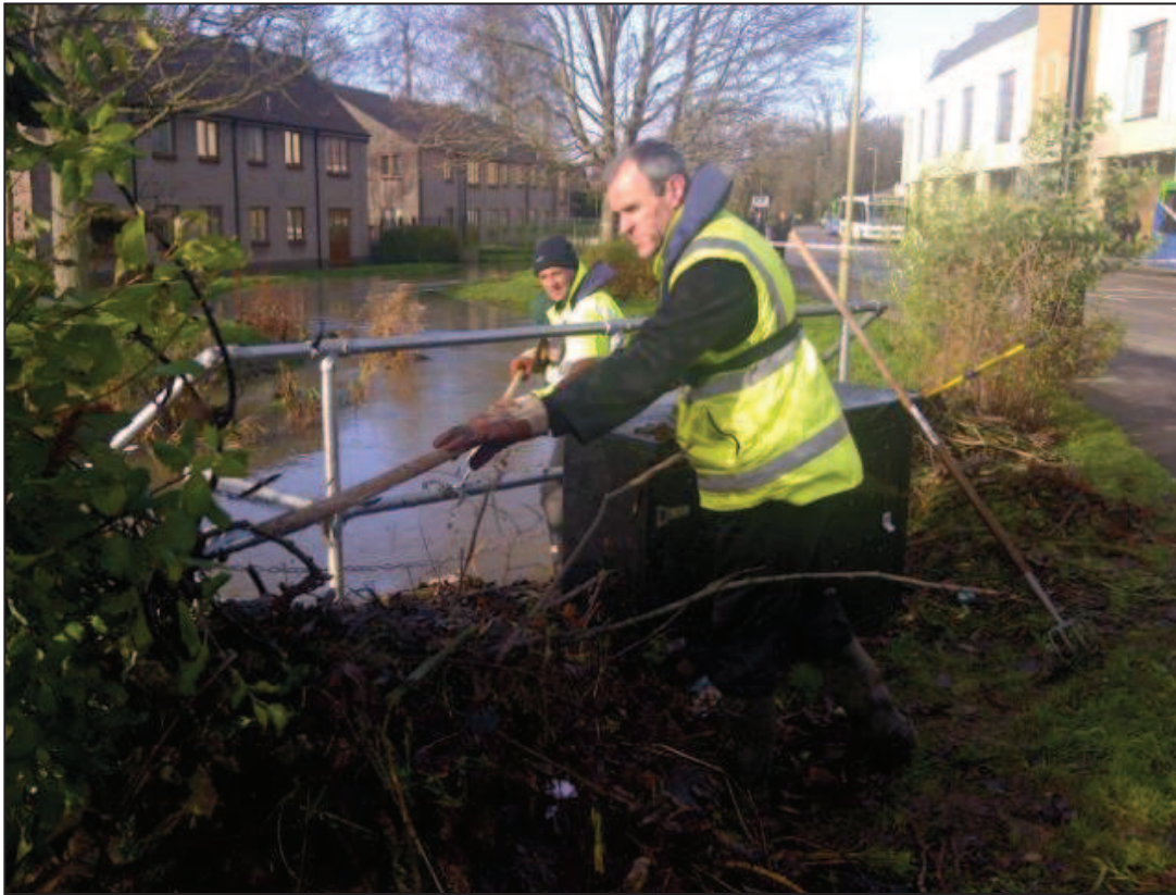
Figure 9: Environment Agency operational team removing debris from the River Bure trash screen at Hanover Gardens
